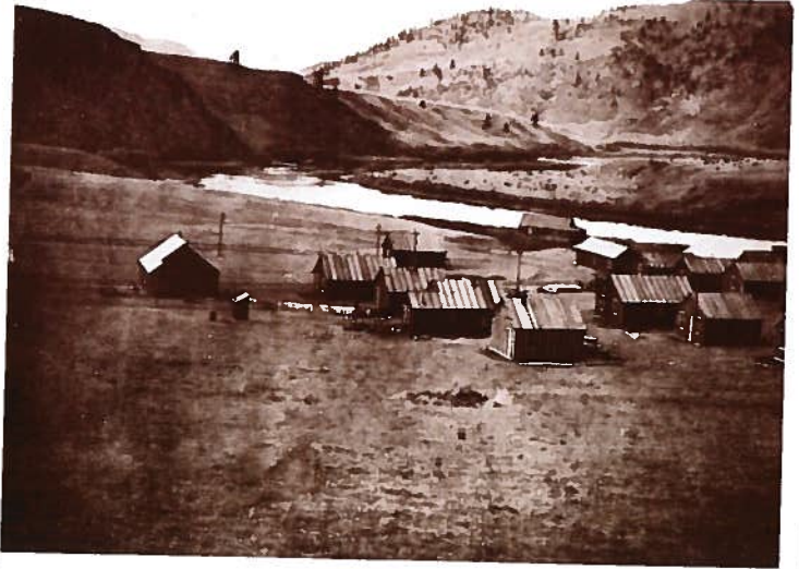
The construction camp at Holter included 115 buildings or structures.
